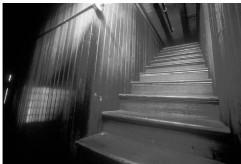
Stair leading to the ceiling
